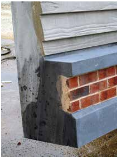
The precaster had to ensure each finish was contained with no spillover as the various textures were cast in the panels. Photo: The Shockey Precast Group.
