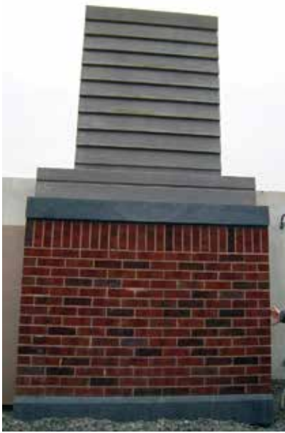
Panels often had more than one texture in them to reduce piece counts. The dividers in openings, which offered a woodgrain appearance, added depth and a window-like appearance but required special attention during transportation. Photo: The Shockey Precast Group.
